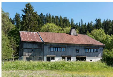
Façade nord. Phot. Sonia Dourlot IVR43_20172500777NUC4A
