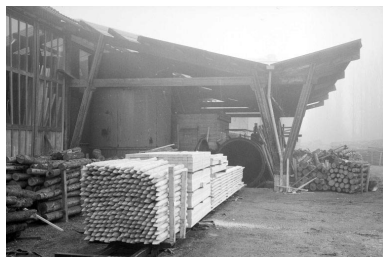
Autoclave. Phot. Laurent Poupard IVR43_19893900277Z
