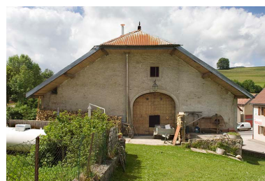
Façade postérieure. Phot. Jérôme Mongreville IVR43_20092500787NUC2A
