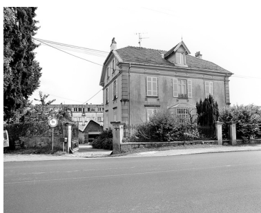
Logement patronal. Phot. Yves Sancey IVR43_19999000317X
