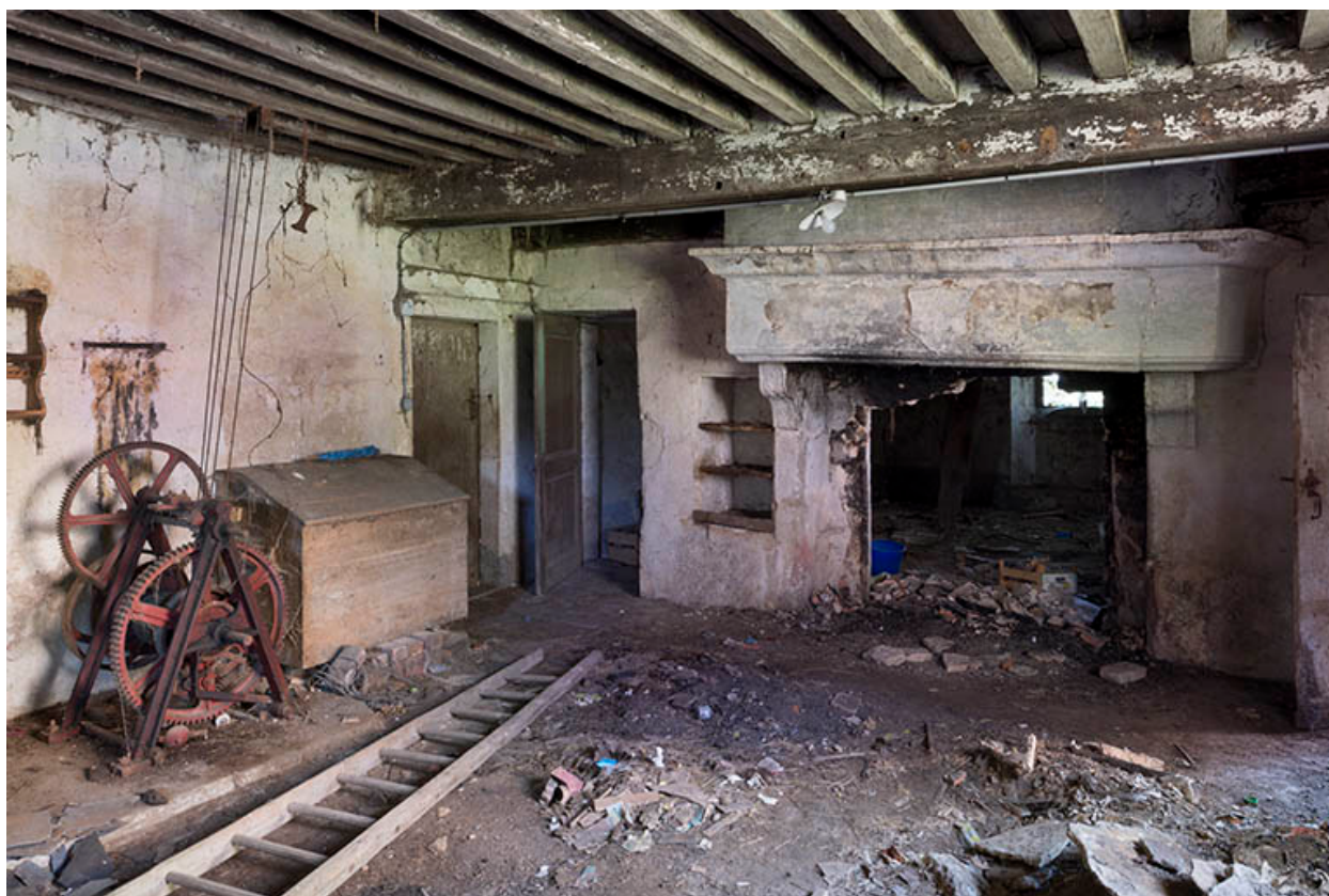
Rez-de-chaussée, logis 16e siècle.
