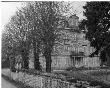
Façade principale. Phot. Jérôme Mongreville IVR43_19853900140X
