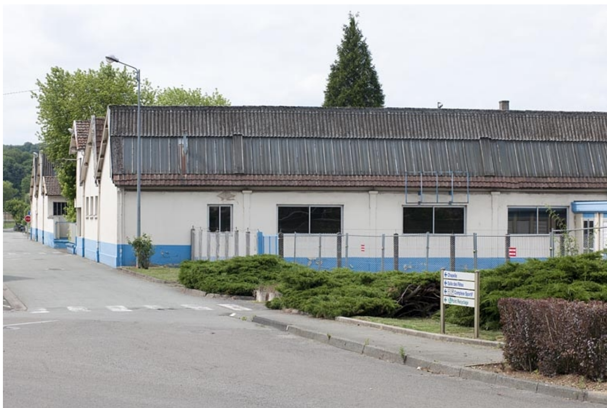
Ateliers de fabrication originels.
