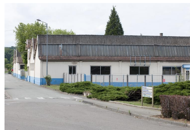
Ateliers de fabrication originels.
