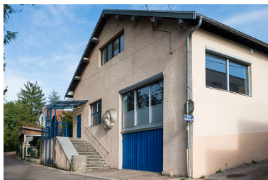
Mur-pignon ouest. Phot. Jérôme Mongreville IVR43_20172501137NUC4A
