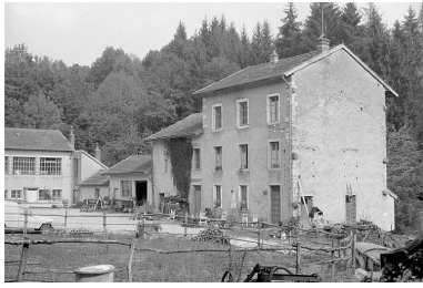
Logement patronal. Phot. Laurent Poupard IVR43_19913901104Z
