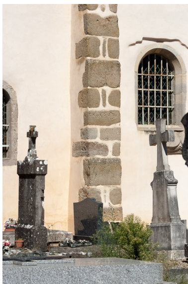
Contrefort de la nef. Phot. Pierre-Marie Barbe-Richaud IVR26_20167100073NUC2A
