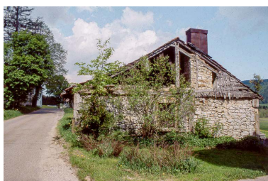
Face droite. Phot. Yves Sancey IVR43_19993900187ZA
