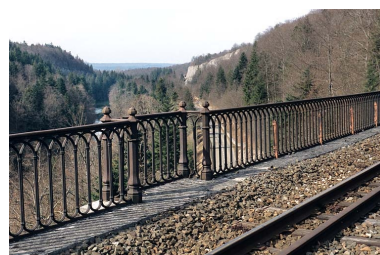
Refuge et garde-corps. Phot. Yves Sancey IVR43_20053900103ZA
