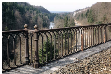
Garde-corps. Phot. Yves Sancey IVR43_20053900101ZA
