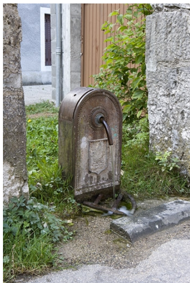
Borne fontaine au 12 rue Emile Zola. Phot. Yves Sancey IVR43_20093900115NUC2A
