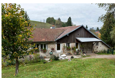
Moulin et logement : façade est. Phot. Sonia Dourlot IVR43_20172501645NUC4A
