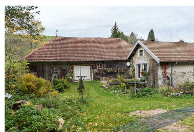
Scierie : façade est. Phot. Sonia Dourlot IVR43_20172501646NUC4A
