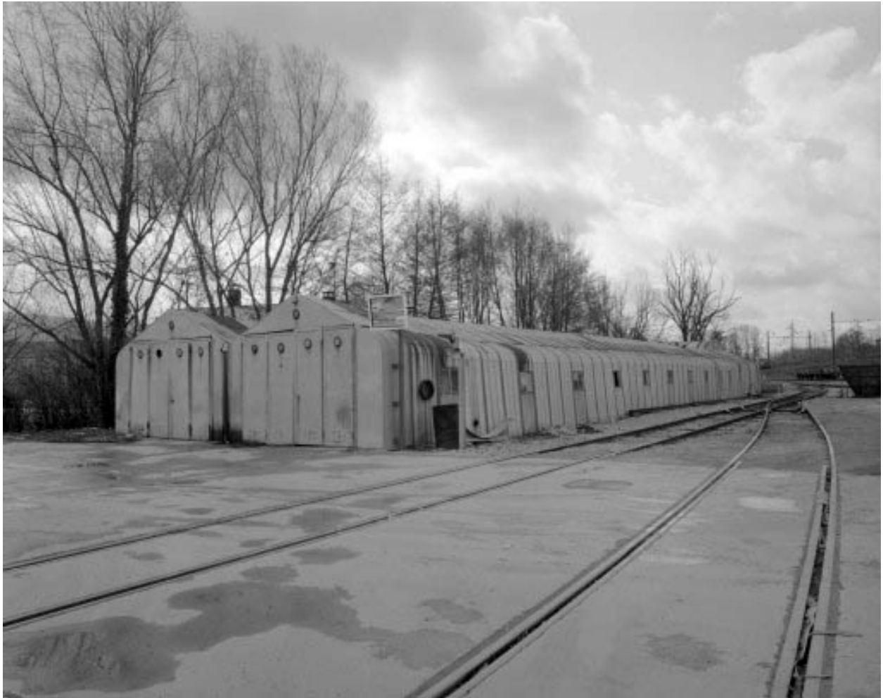
Baraques de chantier (F).
