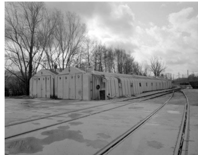
Baraques de chantier (F). Phot. Yves Sancey IVR43_19943901660X
