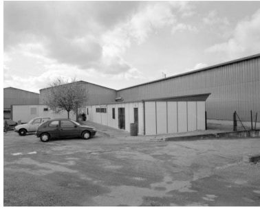
Bungalow (A). Phot. Yves Sancey IVR43_19943901651X
