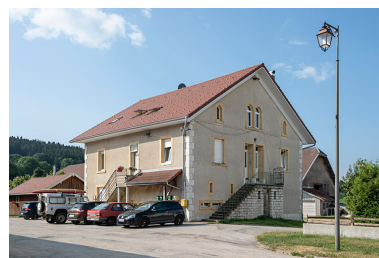
Façades nord et est. Phot. Sonia Dourlot IVR43_20192500641NUC4A
