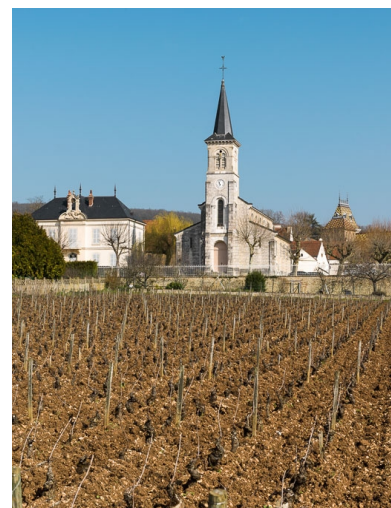
Façade. Phot. Pierre-Marie Barbe-Richaud IVR26_20162100009NUC4A
