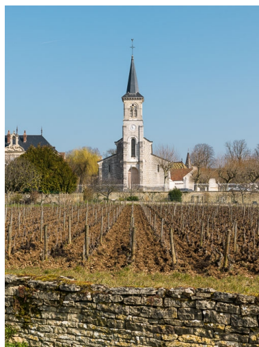
Façade. Phot. Pierre-Marie Barbe-Richaud IVR26_20162100008NUC4A
