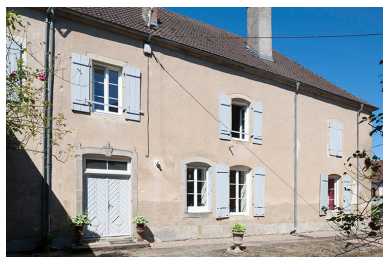
Vue générale, façade est. Phot. Jérôme Mongreville IVR43_20167001079NUC4A
