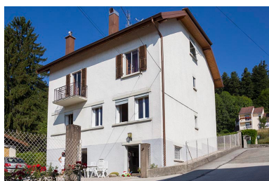
Elévations sud et est. Phot. Yves Sancey IVR43_20132501816NUC2A
