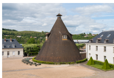
Elévation sud. Phot. Pierre-Marie Barbe-Richaud IVR26_20257100254NUC4A
