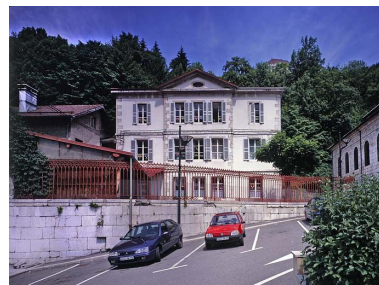
Façade antérieure. Phot. Yves Sancey IVR43_20033900824VA
