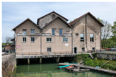
Murs-pignons ouest. Phot. Jérôme Mongreville IVR43_20152501283NUC4A
