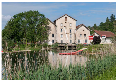
Murs-pignons est. Phot. Jérôme Mongreville IVR43_20152501288NUC4A
