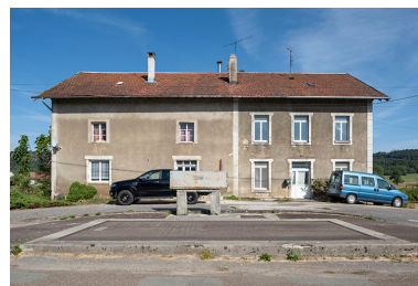
Façade antérieure. Phot. Sonia Dourlot IVR43_20192500651NUC4A
