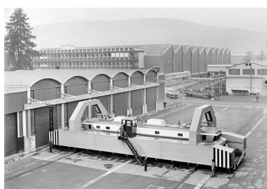
Transbordeur de locomotives. Phot. Jérôme Mongreville IVR43_20029000184X
