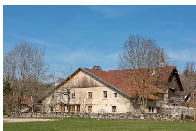
Façade sud, de trois quarts droite. Phot. Sonia Dourlot IVR43_20192500337NUC4A
