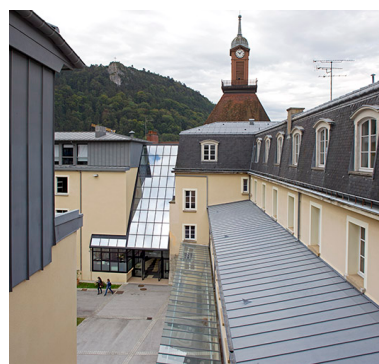
Aile Ouest : toitures at auvents. Phot. Sonia Dourlot IVR43_20143900712NUC2A
