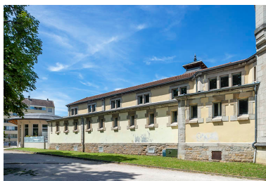
Aile orientale. Phot. Jérôme Mongreville IVR43_20223900768NUC4A
