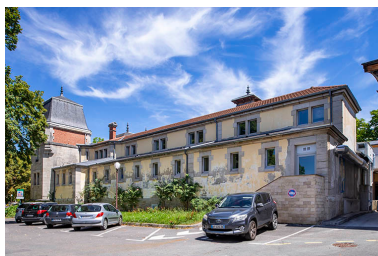
Aile occidentale. Phot. Jérôme Mongreville IVR43_20223900771NUC4A
