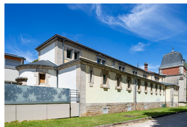
Aile orientale. Phot. Jérôme Mongreville IVR43_20223900769NUC4A
