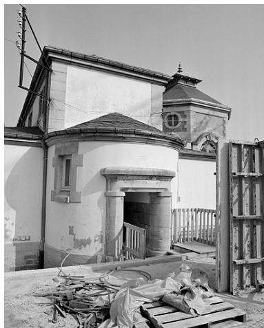
Aile orientale (1983). Phot. Yves Sancey IVR43_19833900095X
