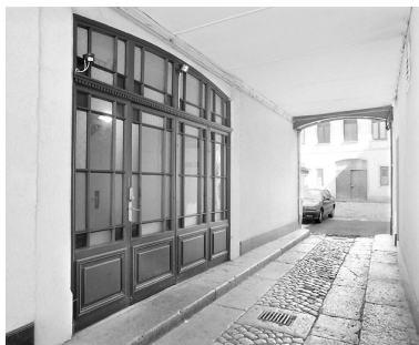
Passage couvert. Phot. Yves Sancey IVR43_20033900724X
