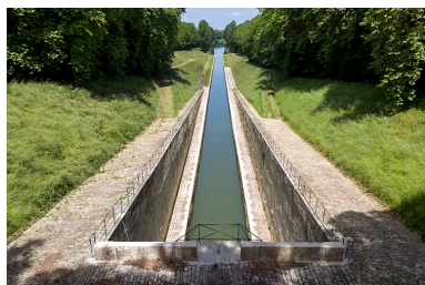
Le canal de navigation, vue amont. Phot. Sonia Dourlot IVR43_20157001007NUC2A
