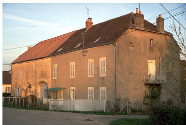
Magasin industriel, grange, logement patronal. Phot. Laurent Poupard IVR43_19883900666ZA
