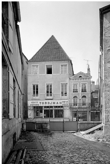
Façade antérieure de face. Phot. Yves Sancey IVR43_19897000116V
