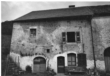
Partie habitation. Phot. F. Pernin IVR43_19743900163Z
