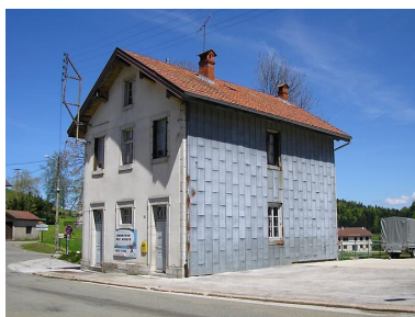
Ecole. Phot. Marie-Pierre Reynet IVR43_20083900365NUC1A
