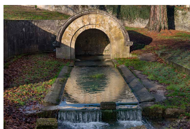
Bassin. Phot. Jérôme Mongreville IVR43_20197000145NUC4A
