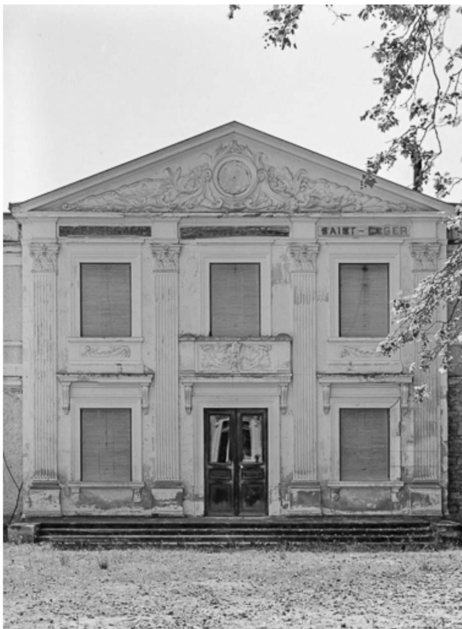
Façade antérieure, avant-corps.
