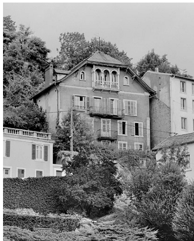
Façade principale. Phot. Jérôme Mongreville IVR43_19872500780X
