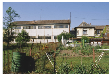
Façades nord. Phot. Yves Sancey IVR43_20009000538ZA
