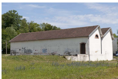
Magasin industriel est. Phot. Jérôme Mongreville IVR43_20112501186NUC4A
