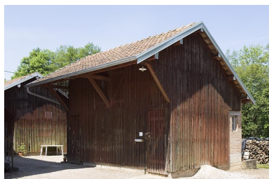
Bûcher. Phot. Jérôme Mongreville IVR43_20097000315NUC2A
