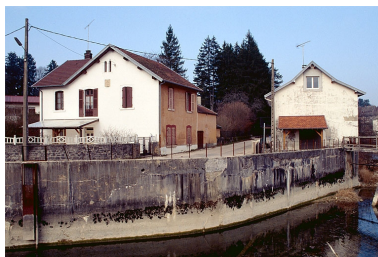
Logements. Phot. Jérôme Mongreville IVR43_19963900053ZA
