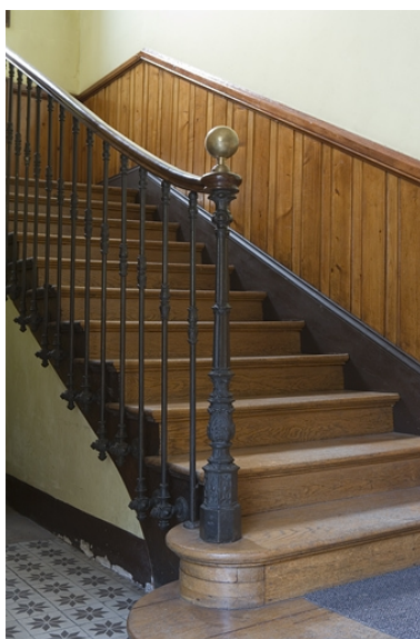
Escalier. Phot. Yves Sancey IVR43_20093900129NUC2A
