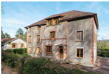
Façade principale. Phot. Pierre-Marie Barbe-Richaud IVR26_20195800222NUC4A
