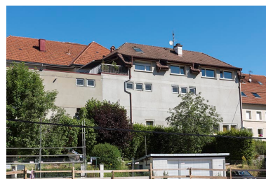
Façade sud. Phot. Sonia Dourlot IVR43_20162501385NUC4A
