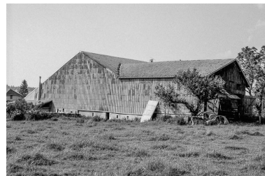
Façade postérieure. Phot. Gilbert Poinot IVR43_19752500782Z
