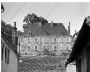
Façade postérieure, de face. Phot. Yves Sancey IVR43_19897000408X
