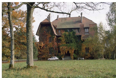
Façade ouest. Phot. Yves Sancey IVR43_20009000823ZA
