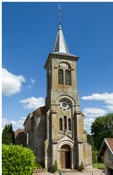
Façade principale. Phot. Sonia Dourlot IVR43_20157001030NUC2A
