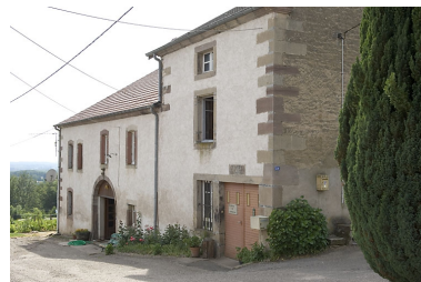
Logement, parties agricoles et chai. Phot. Jérôme Mongreville IVR43_20077000138NUCA
