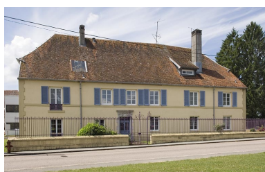
Logement patronal. Façade est. Phot. Jérôme Mongreville IVR43_20097000539NUC2A
