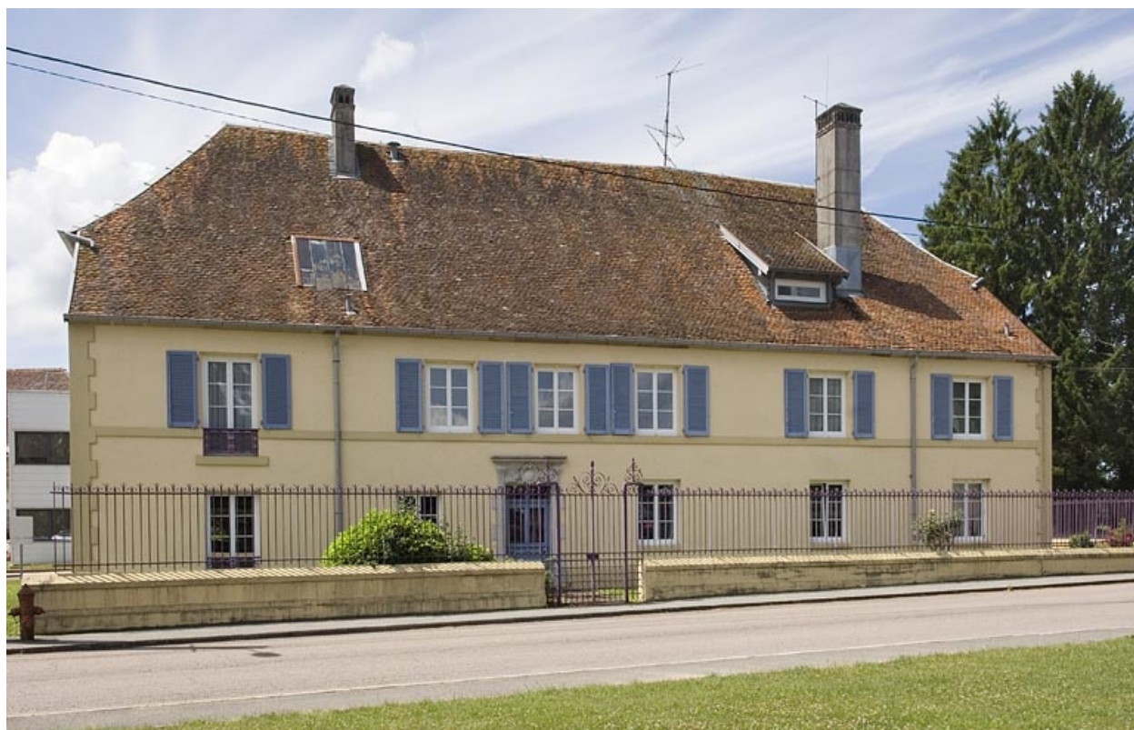
Logement patronal. Façade est.
