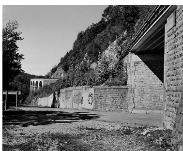
Elévation sud, de profil. Phot. Yves Sancey IVR43_20053900357X
